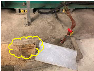
Exposed fuel pipes
