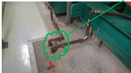
Emergency Generator HS5 (Stand on 200mm-thick concrete plinth)
