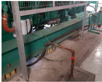
Fuel pipes to/from fuel tank and the generator
