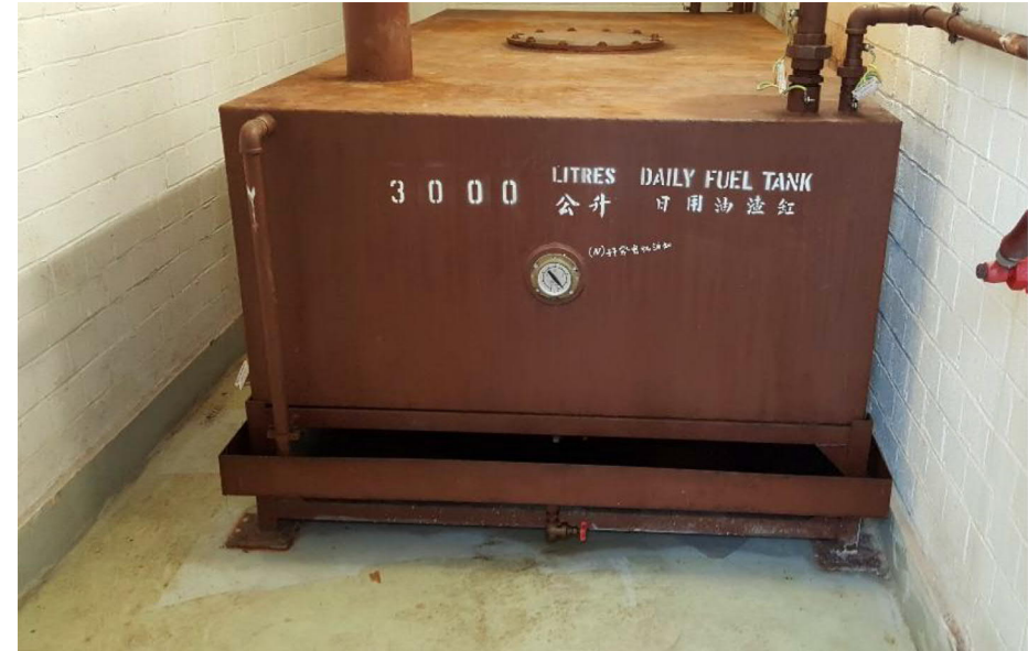
BH9 View 1 - 3000L Above-ground Fuel Tank (BH9)
