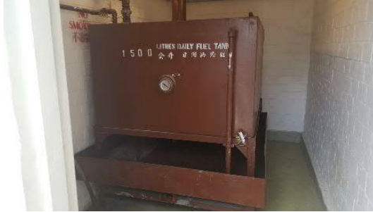
1,500 L fuel tank (HS4) with metal drip tray
