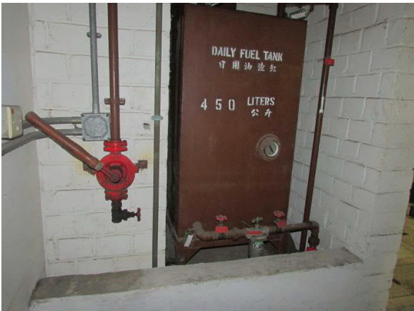
BH7 View 1 - 450 L Above-ground Fuel Tank
