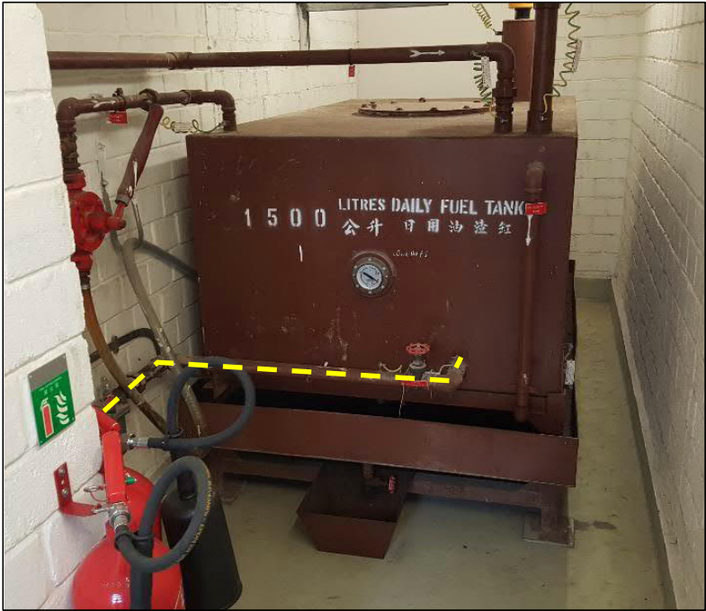
1,500L fuel tank (BH10) with metal drip tray
