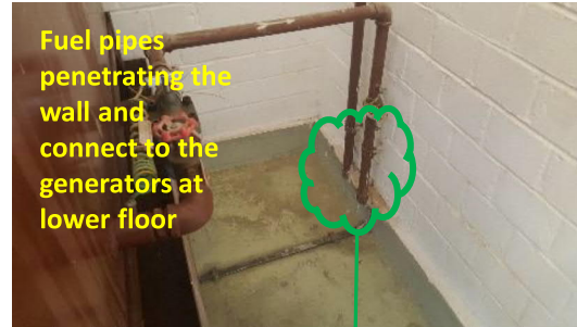
Fuel pipes penetrating the wall and connect to the 1500L fuel tank at upper floor
